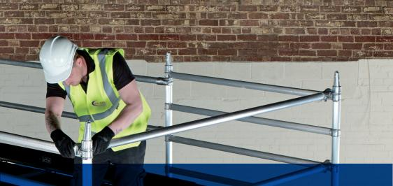
The maximum base dimension is 6.10m x 3.2m accommodating several operatives but smaller base sizes can be built by using alternate sizes of tower and link beams. It is strongly advised that a maximum platform height of The Boxing Ring is 4.2m. There are many smaller platform heights available.
